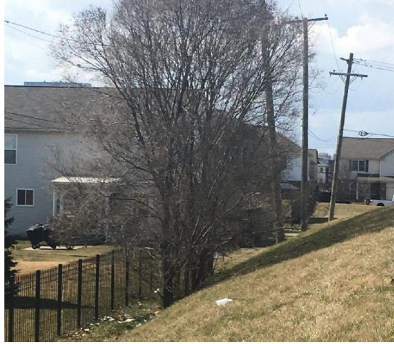
South Side of Berm
